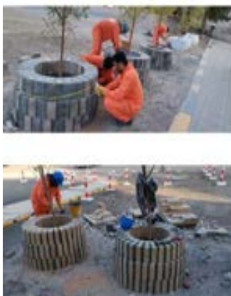
WASTE KILN BRICKS RE-USE
